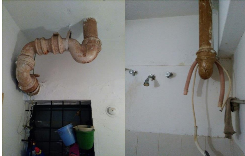
Image 8: Exposed Pipes inside the House
