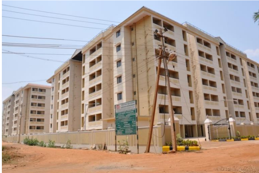
Image 1: View of the High rise apartment- KHB Heritage
